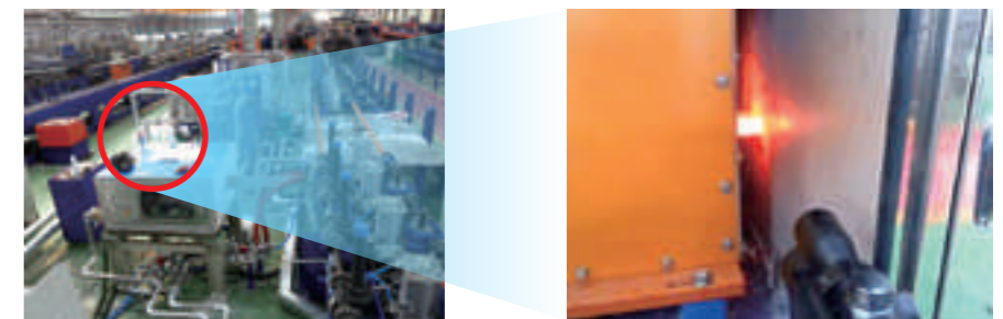
Seamless Pipe Heater & Quenching equipment
